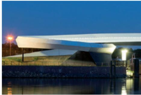
across the harbour entrance and terminates in a circular ramp. The complex geometry of the superstructure required construction of a 3D model on which the workshop drawings were based. The steel superstructure was manufactured and delivered to site in sections. The 70 m long and approx. 200 tonne heavy section of the bridge across the harbour entrance was positioned using a floating crane and assembled on the land side, parallel to the harbour basin.
